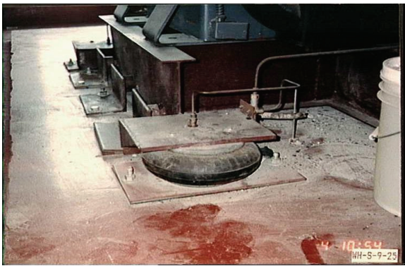
Figure 2. Chiller shifted from rubber pad isolation mount (EPRI)
